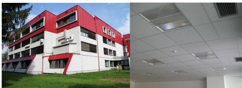
Figure 6 & 7: View of the renewed facade and the internal features, with relevance with internal lights and airflow system.
