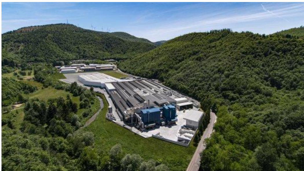
Figure 4: View of Vetreria Etrusca Plant with solar panels on the roof and the 38000 trees wood around it
